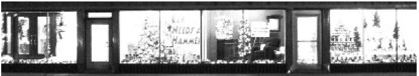
Niehaus has dressed the windows in the old Ford Building to celebrate the Holidays in grand style.
