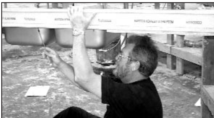
Steve Lanning - installing sink to finished laminate counter top.
