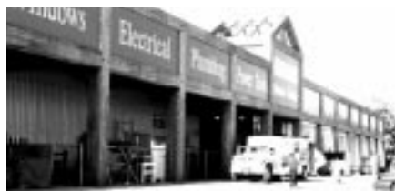
Niehaus Home Center - Remodeled in 1996
